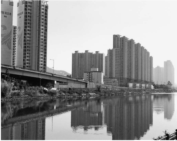
Fig. 2 Apartment complexes on the Nakdong River in Busan, South Korea. Photograph by Nicholas Albrecht, December 2011.
